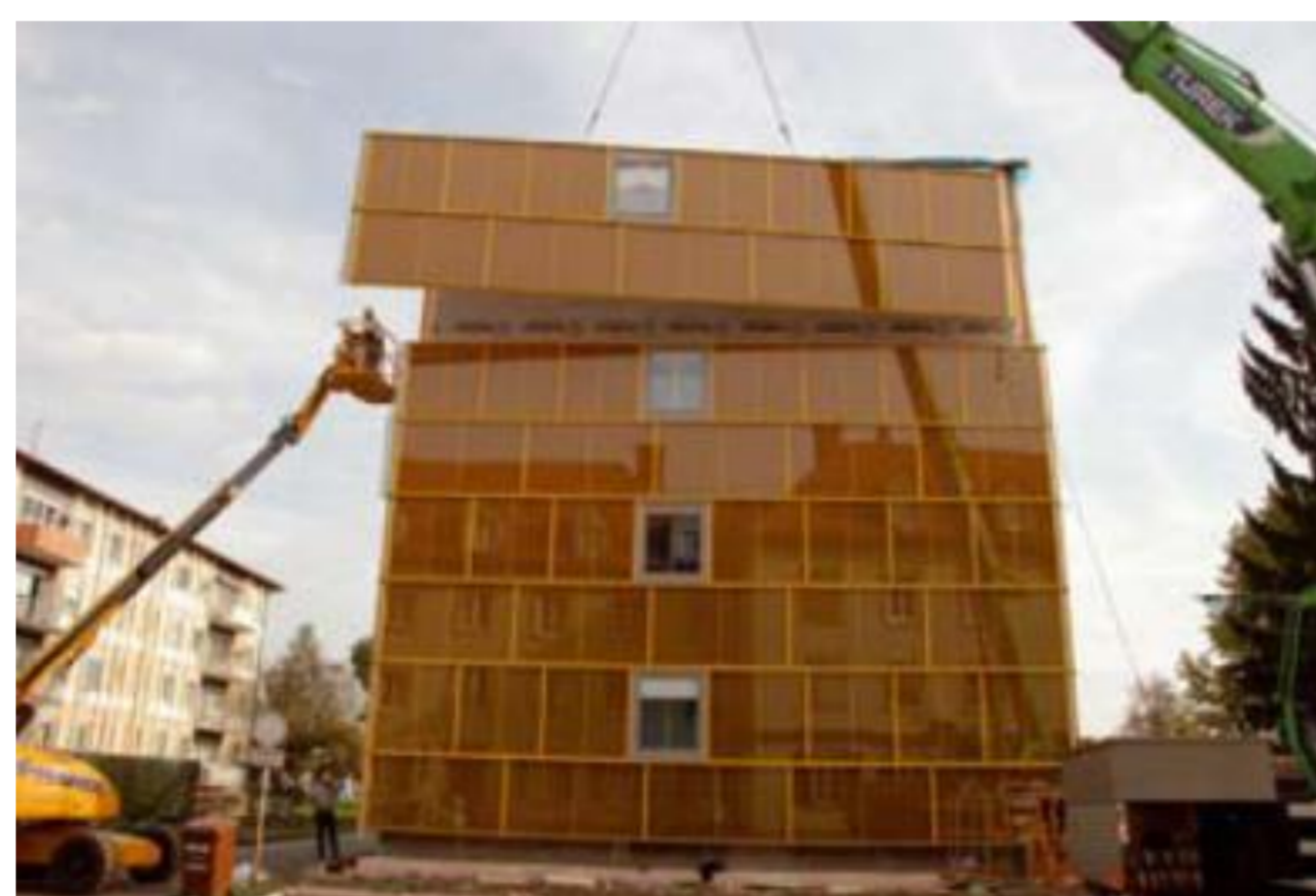
Pre-fabricated multi-active façade in Vienna
