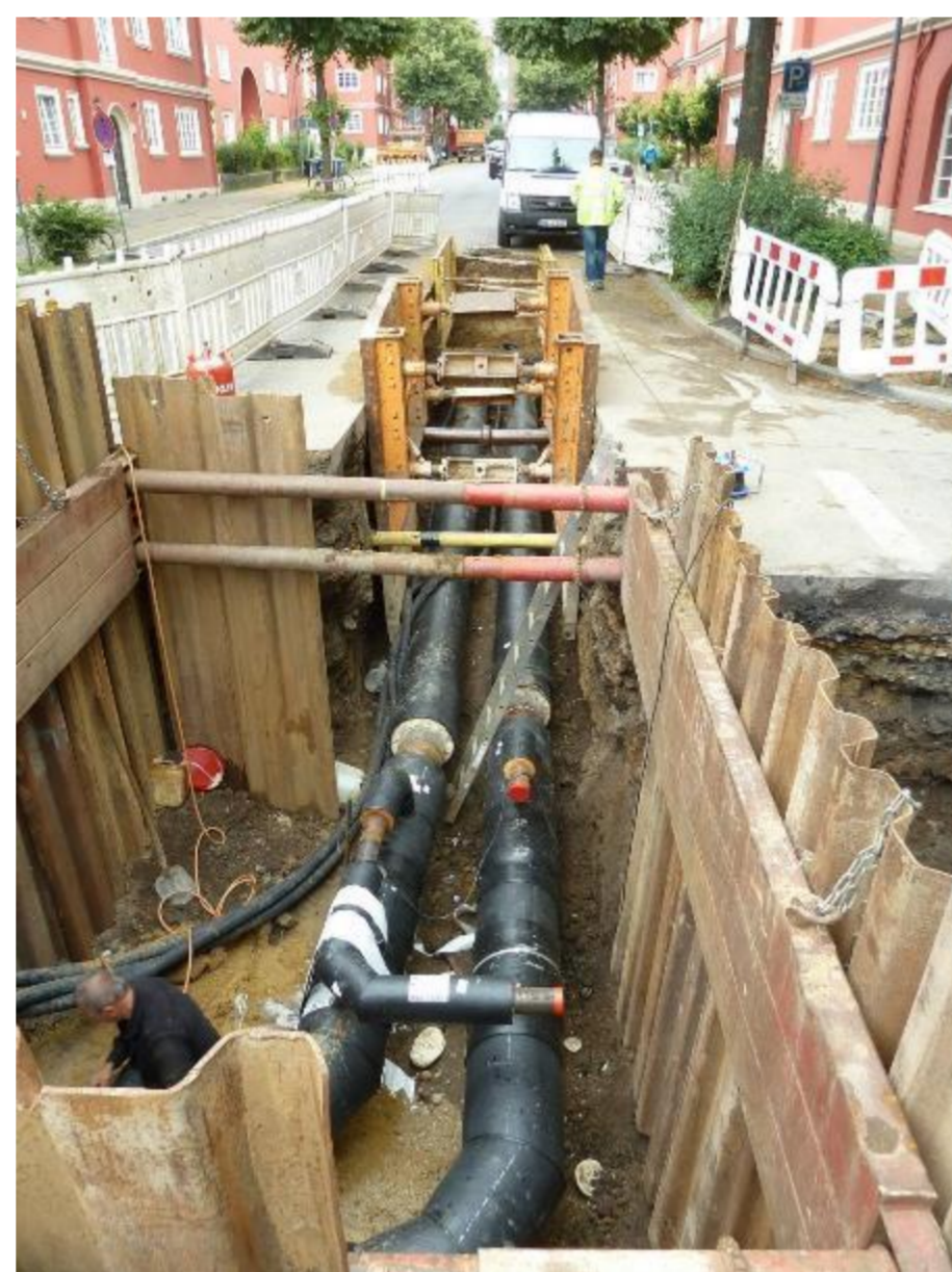
Heat Recovery from the Sewage water in Aachen
