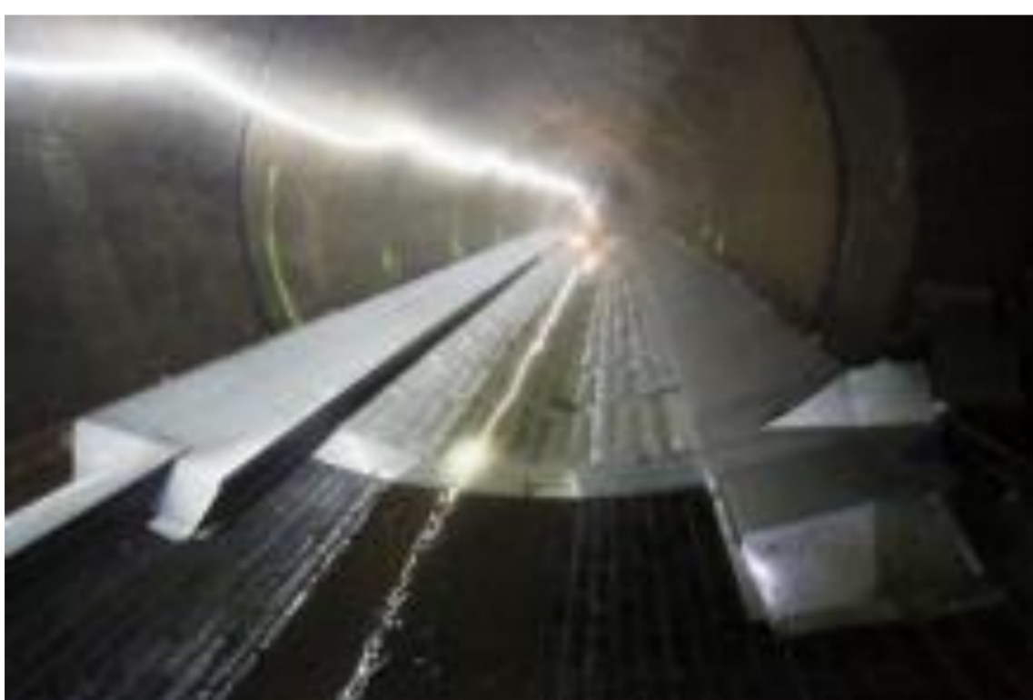
Heat Recovery from the Sewage water in Aachen
